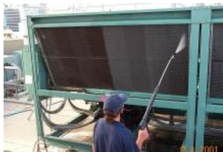
Unit being pre-treated before the coating process can commence.
